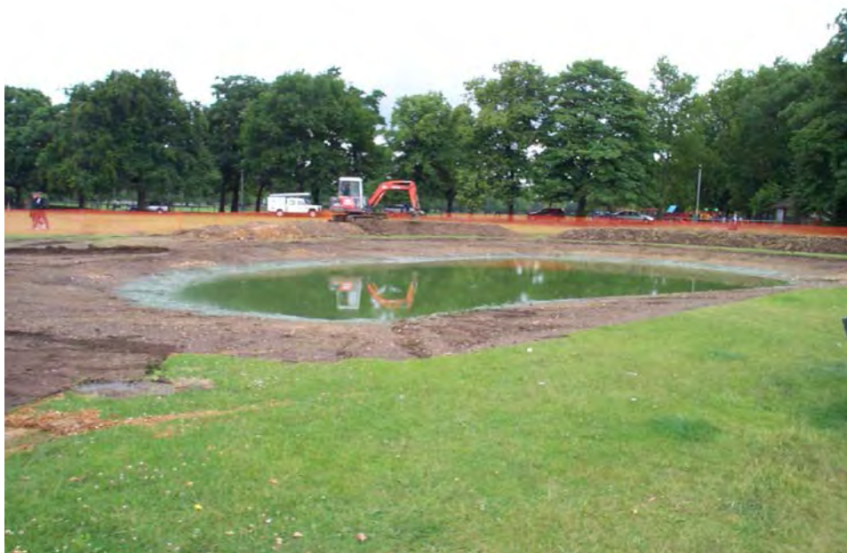
Figure 66. Creating a new surface and flood water storage area next to Eagle Pond, Clapham Common, Spring 2004 (London Borough of Lambeth)
