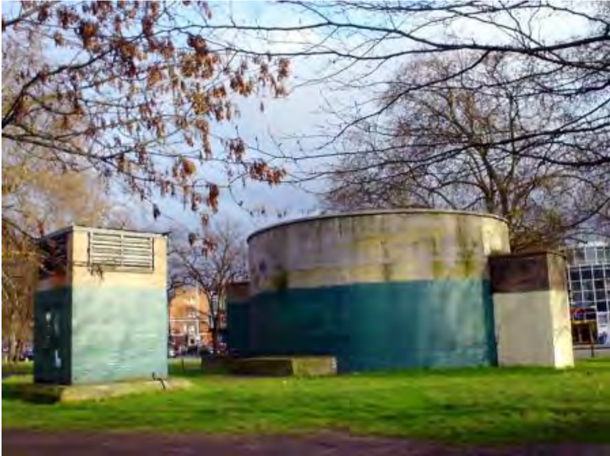
Figure 74. Exterior view of the Deep Level Air Raid Shelter on Clapham Common, showing the central 'Rotunda' and ancillary buildings (London Borough of Lambeth)
